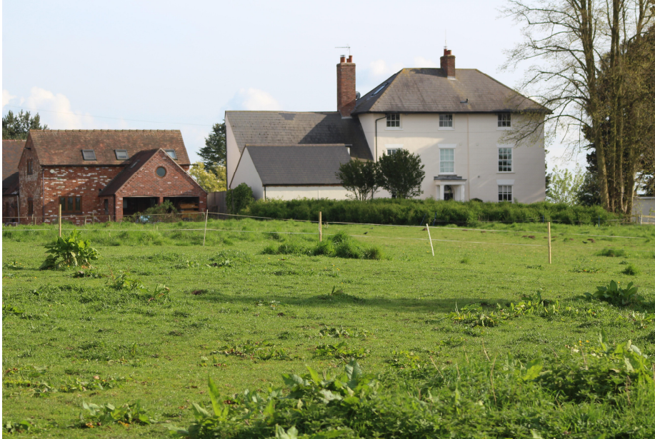
Looking across Site 272 to Dunsley House in the Kinver Conservation Area
