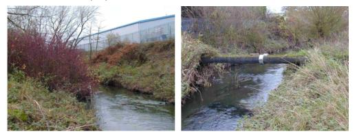
STW have advised that the most eastern pipe crossing is redundant, so this could possibly be removed, though this would need to be agreed with STW. The other pipe crossing consists of a sludge transfer main from Cannock STW to Four Ashes STW. These will need modifying in an agreed manner to allow for navigation beneath.
