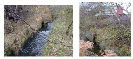
Joveys Lock appears to be of a standard brick construction. The brickwork appears to be in a poor state of repair and as a minimum would require repointing and rebuilding. Again as with the previous existing lock, the gates have been removed. A detailed survey of the lock would be required to determine if it is at the correct level or structurally viable to be used as part of the restored canal.
