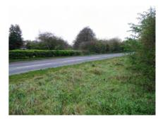
The first option considered would maintain the water level of the canal close to that of the existing level and would require the road surface level of the Straight Mile to be raised by approximately 2.8m. However, this is not considered feasible because of the length and height of the approach embankments required, which would force considerable reconfiguring of the adjacent junctions and accesses as well as severe visual intrusion for the adjacent householders.
