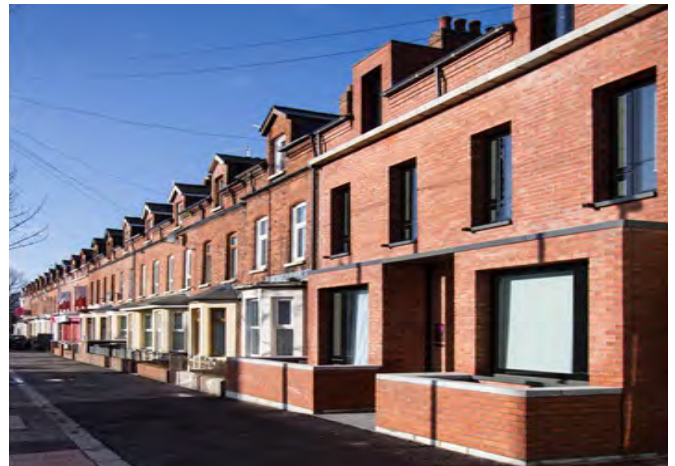
This modern infill development respects and continues the rhythm of the existing street.
