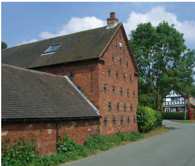
This successful barn conversion retains the original brick detailing whilst simple roof lights have been used to bring light into the building without compromising the traditional form.
