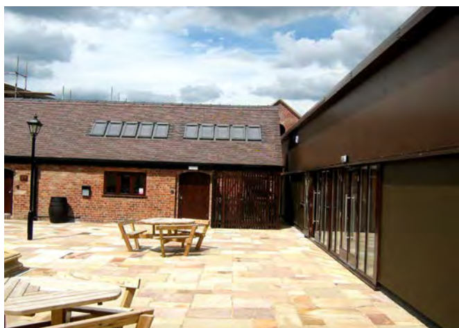
Building layout may take inspiration from agricultural-style arrangements such as this conversion of a former agricultural complex at Dunston Business Park.
