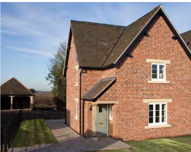
Burnhill Green is a high quality development in a rural context. Red bricks, traditional lime mortar and reclaimed roof tiles tie the development to its local context. Consideration of the appearance of the design and consultation with the local community result in a development which maintains the character of the local area.
