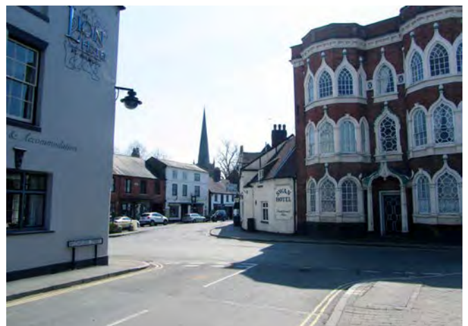
An example of an historic church steeple in Brewood remains clearly visible in the village street scene.
