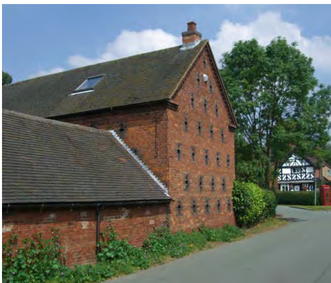
This successful barn conversion retains the original brick detailing whilst simple roof lights have been used to bring light into the building without compromising the traditional form.
