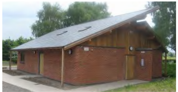
The simple style and low height of the Highgate Common Visitor's Centre sits well in its surrounding landscape. An interesting roof style allows windows to be added into the stepped elevation without compromising the simplicity of form.
