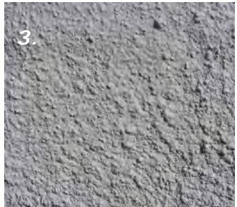
3. Rendered surfaces on the District's historic buildings were painted in a limewash, limited to a range of colours including cream, near white or stone. Brighter and pastel colours are not widely found.
