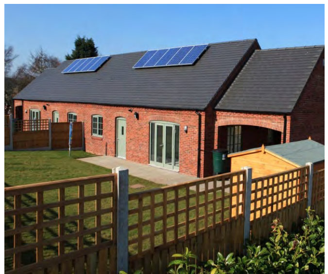
This development on Himley Lane, Swindon, uses the traditional farmstead layout - common in South Staffordshire - whilst creating contemporary homes with high energy performance and modern materials.
