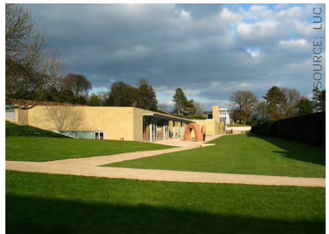
This building at the Yorkshire Sculpture Park is set into the hillside and below the tree canopy of the surrounding woodland. The green roof of the building in combination with carefully placed hedge and grassed areas blends the building seamlessly into the surrounding landscape from elevated viewpoints.
