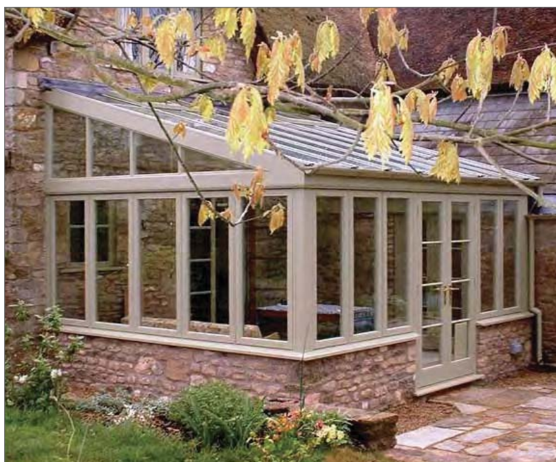
Conservatories should complement the original building
