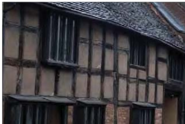
A typical timber-framed building
