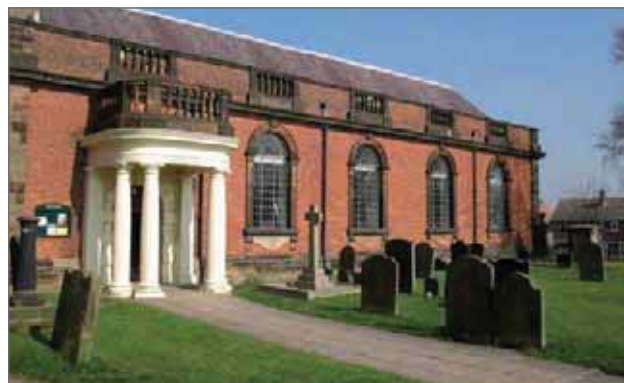
Successful and subtle repair at Shareshill Church
