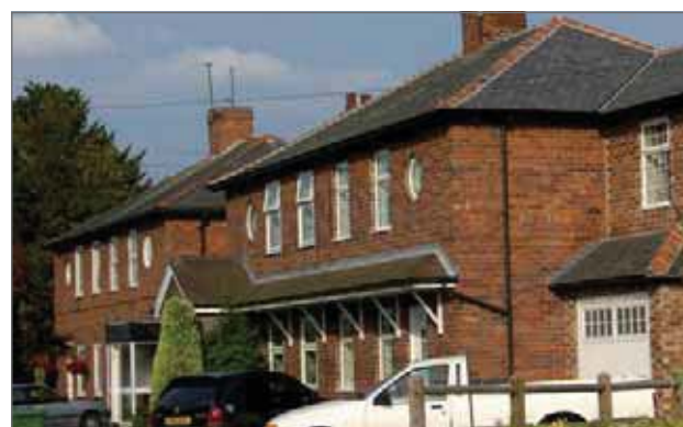
Consistent material choice which is in keeping with existing architecture
