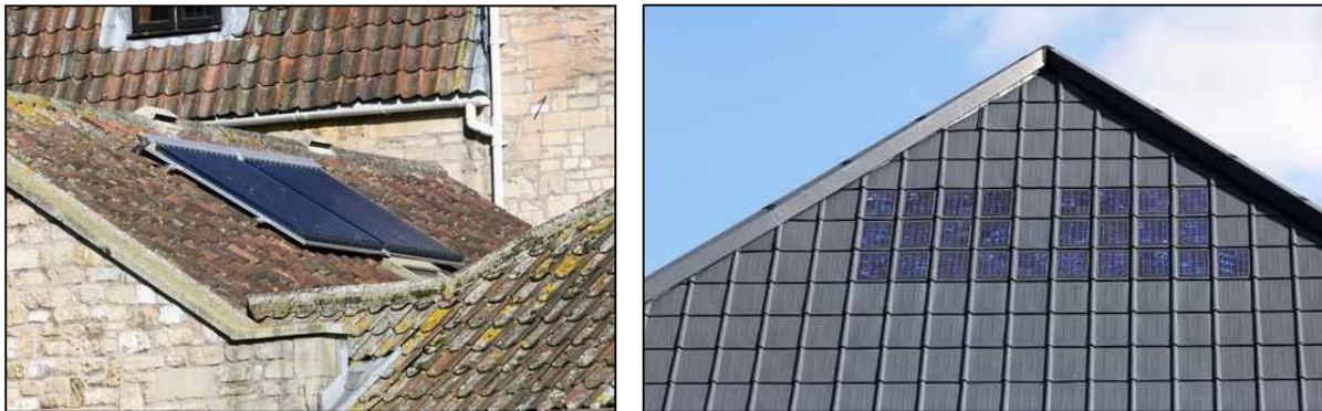
Figure 3: a) Discreetly located solar panels on historic buildings and b) solar roof tiles
