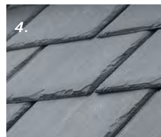
4. Blue-grey Welsh slate is also common across the district. Slate is lighter, more durable and weatherproof than clay. The colour can vary subtly from dark blue/grey to purple/grey.
