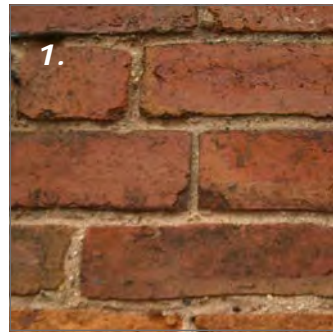
1. The locally occurring Keuper Marl Clay was historically accessible and is widely used in many of the estates and larger villages. The distinctive local brick is red-brown in colour, soft in construction and weathers to produce a rough texture.
