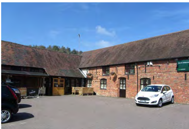
This barn conversion retains the arrangement of buildings looking inward to a central courtyard.
