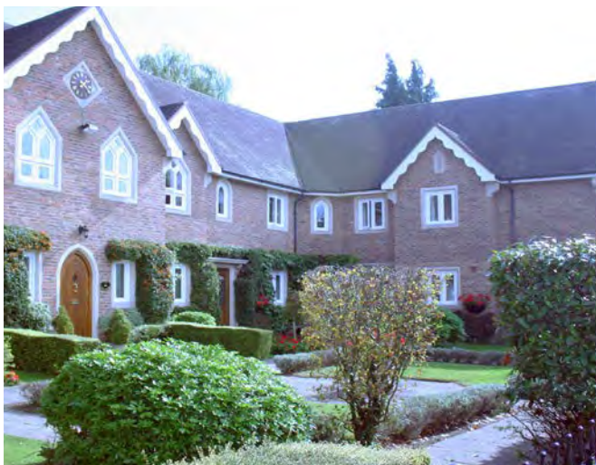
Riverside Court in Kinver has been planned around a central courtyard, setting the building back from the road and creating a community space with natural surveillance from overlooking windows.
