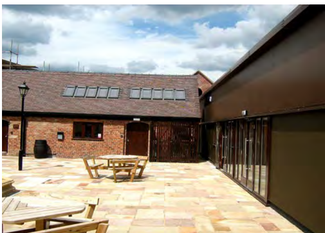
Building layout may take inspiration from agricultural-style arrangements such as this conversion of a former agricultural complex at Dunston Business Park.
