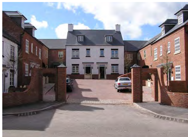
A successful 'Home Zone' achieved with an implied gateway established with local brickwork and a change in surface treatment to identify the shared surface zone.
